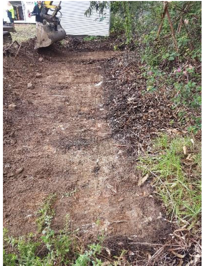
Fig. 31. Trench 1 dug using blade bucket along Sth building line
